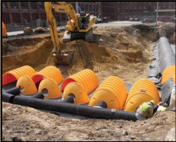
***Installation of a drainage substructure as part of Lawrence Revitalization Project for the Lawrence Community Works.***
