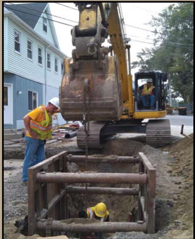
***Crew installing a water gate, part of the water main upgrade portion of the Coburn St. project, Framingham, MA.***
